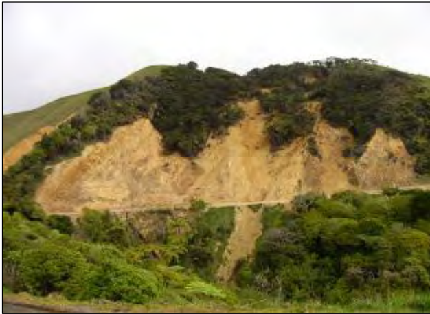
Image3: Land erosion on the Marokopa to Kiritehere road. Shows major slip requiring re-stabilisation. © KCL
