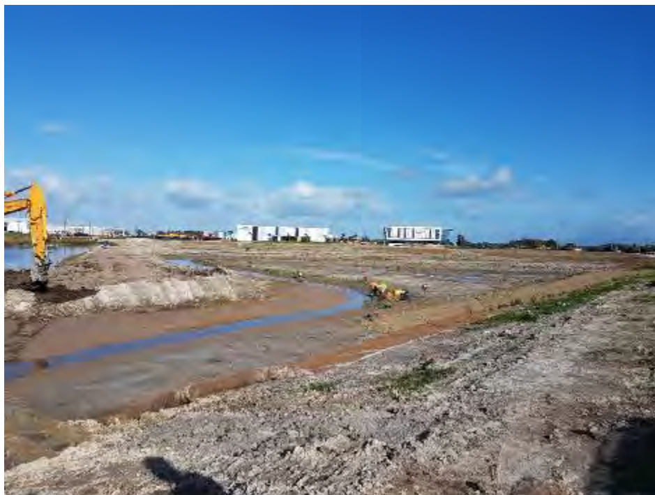
Figure 1 – Photograph showing Porters wetland being planted, 9 th May 2018
