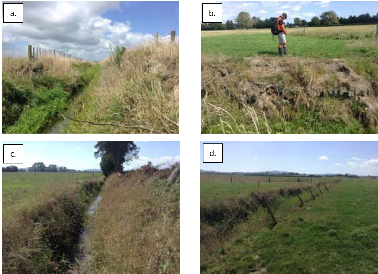
Figure 5: Figure 5a and 5c indicate the typical channel form along reaches 9 and 10 respectively. Figure 5b and 5d illustrate upper bank instabilities along reaches 9 and 10 caused by steep bank angles and poor fence alignment.
