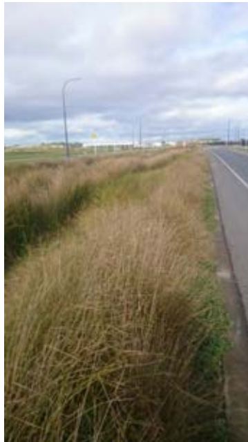
Figure 6-2: Central swale along the main road through the Porters development (looking south)
